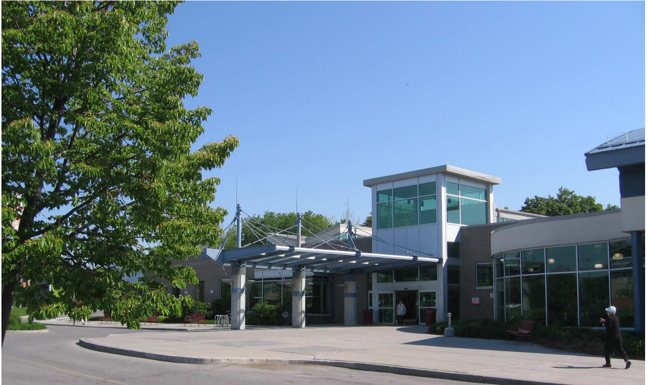
Figure 19-5: Mississauga has many beautiful parks and recreational facilities, such as the Frank McKechnie Community Centre and Library, located in the Hurontario Neighbourhood Character Area. In addition to City reserves, development contributions also play an important role in the creation of open spaces and recreational facilities for all residents to enjoy.
